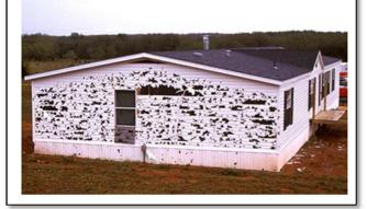
Nonstructural components of one wall have sustained damage.
