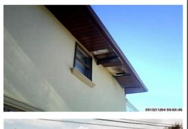
Damage to this soffit represents nonstructural damage to the roof.
