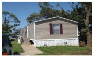
The only damage to this manufactured home is the missing skirting.
