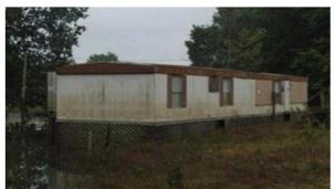
Visible water line above the floor system.
