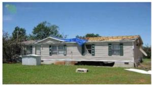
Although much of the roof is missing, the structural ribbing of the roof system is still intact.
