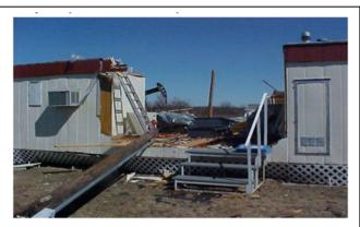
The manufactured home is missing the roof and at least two walls.
