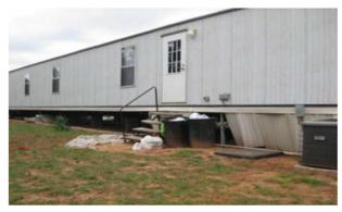
There is no visible water line and only skirting is missing or bent.
